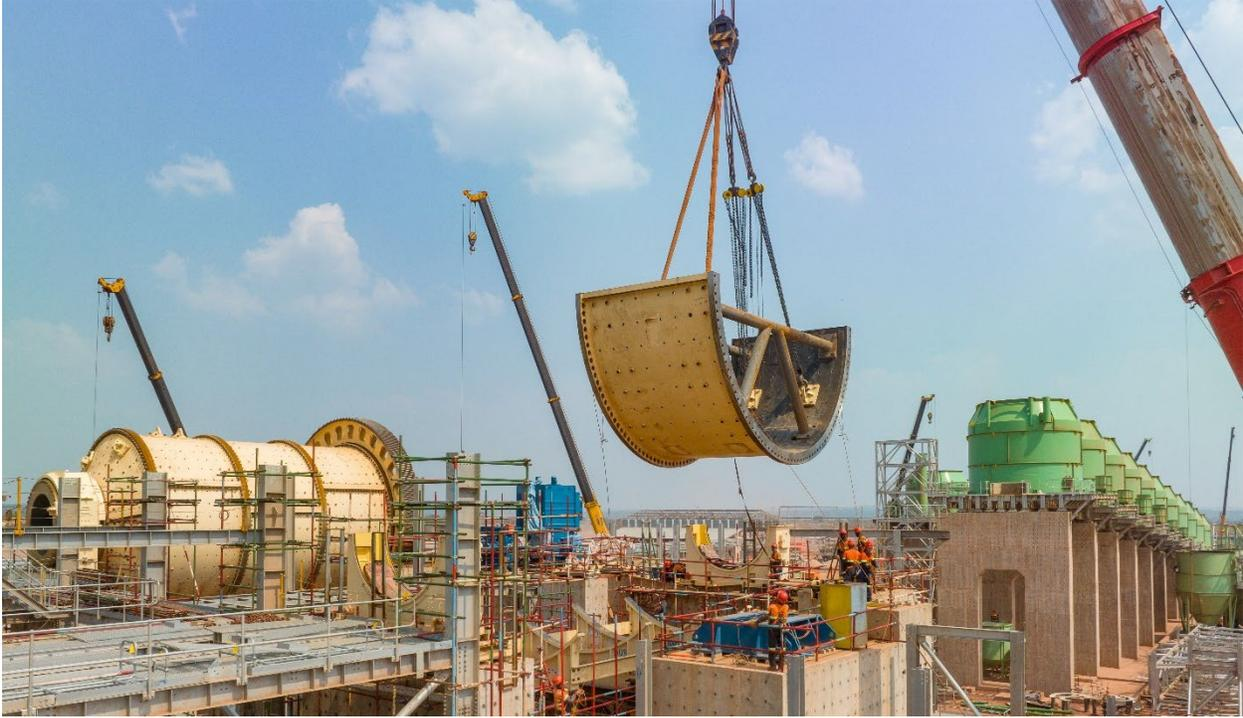
**Construction of the concentrate thickener is progressing well at Kamo-Kakula's Phase 3 concentrator site. The process design of the Phase 3 concentrator is very similar to that of the Phase 1 and 2 concentrators, but 30% larger.**
